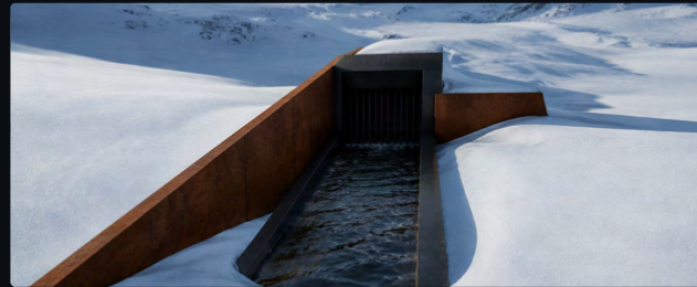
Water intake and treatment
